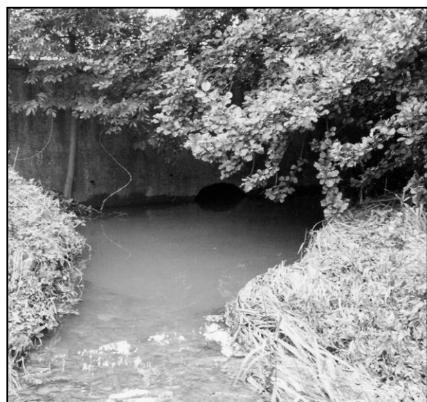
Figure 4 - Photograph of Culvert (1996)
